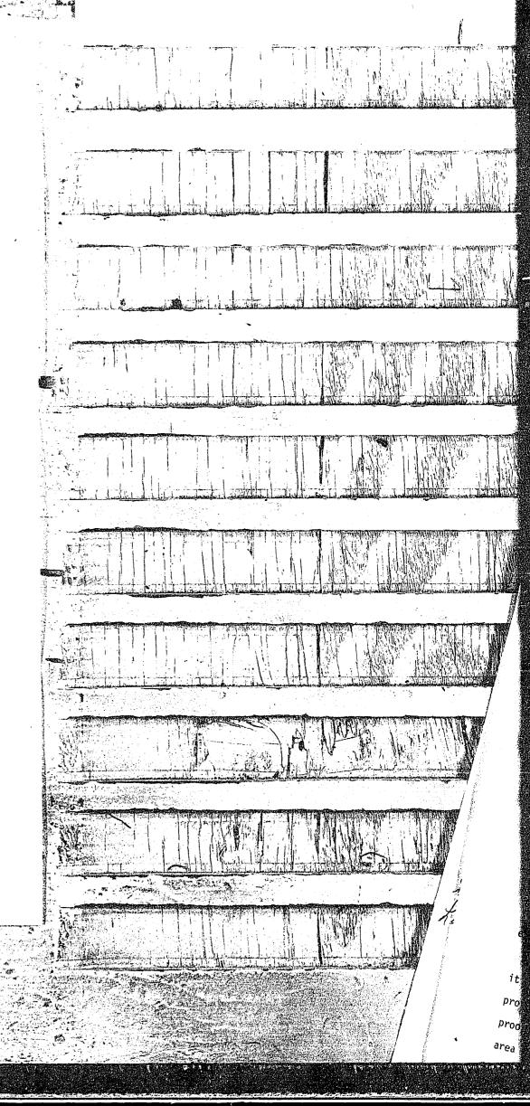
In the fall of 1927 we replaced the headgate in the opening, tearing out our work of the previous spring and made the headgate so we could control water by merely taking boards out or placing them in,
